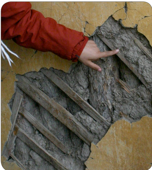
SOVIET ERA WOOD/ADOBE CONSTRUCTION -SMALL DIAMETER LOGS ENCASED IN WOOD LATTICE AND ADOBE LATHE
